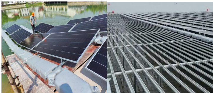
Steel pipe scaffold platform
