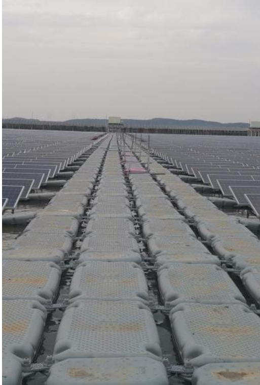
North-south maintenance access walkway
