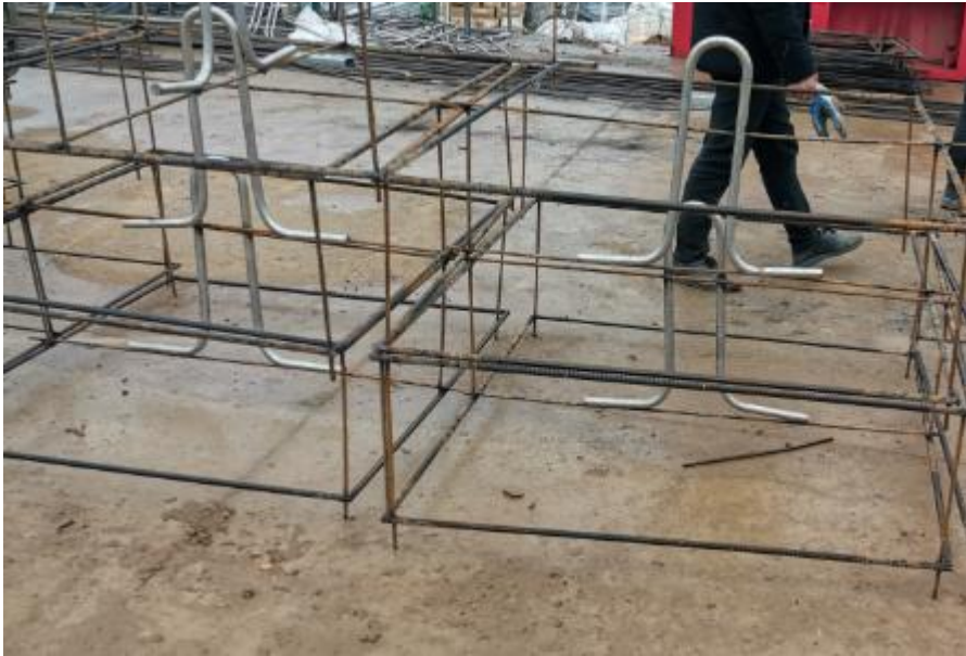
Precast concrete gravity anchor
