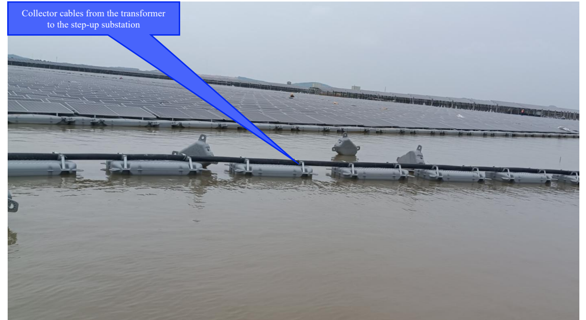
Collector cable laying
