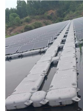
Samll lake-Cable landing and maintenance walkways
