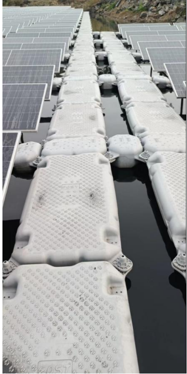
North-south maintenance access walkway
