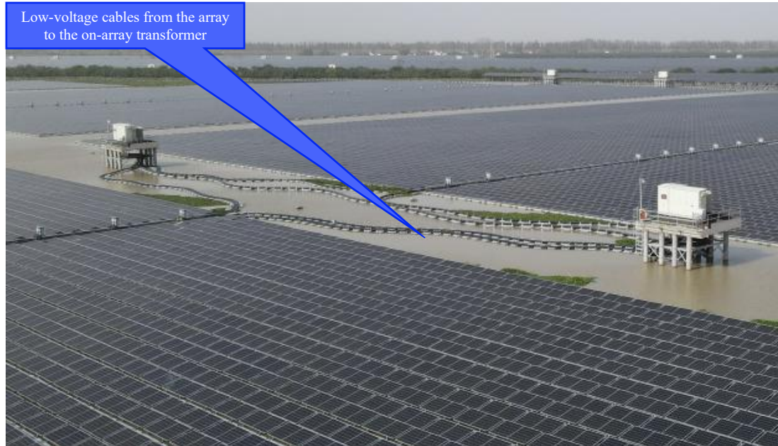
Low-voltage cable laying
