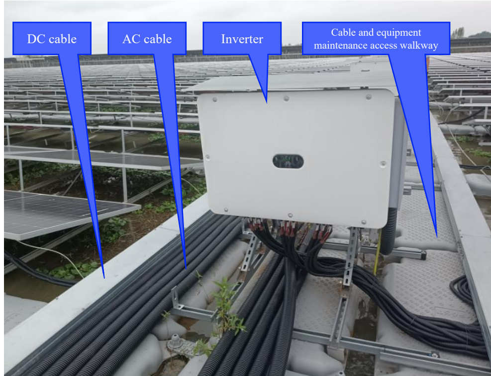
Cable laying and O&M in the central walkway of the floating array
