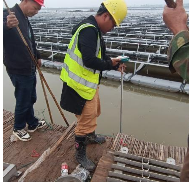
Anchoring foundation positioning
